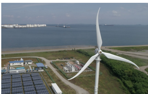
The REIDS-SPORE platform: a microgrid for energy autonomy in isolated sites, here on Semakau Island, Singapore.
